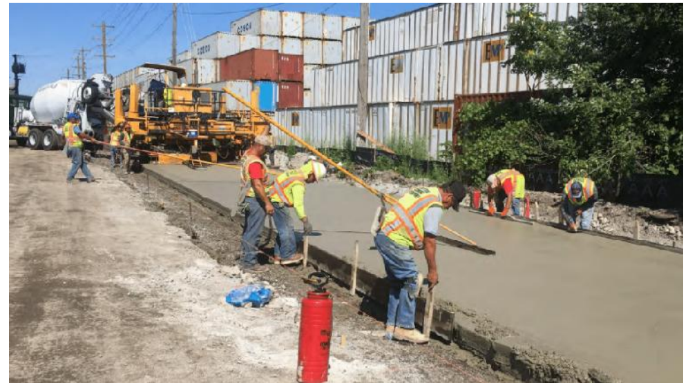
156 th St. Improvements near LB Steel
