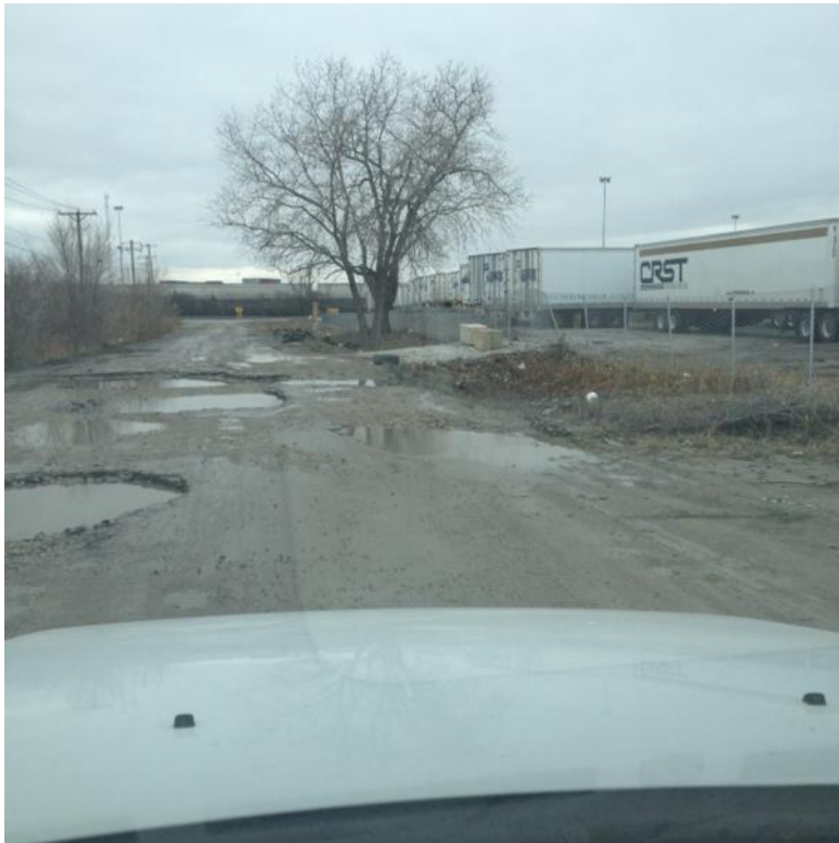
167 th St. Looking West Toward Center St. and CN Intermodal Terminal
